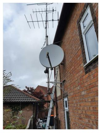
The dish just about fitted there, I was concerned being larger than the previous dish it might not be able to reach 26E without hitting the house, I connected my meter up to the LNB and configured it for the QO-100 beacon on the Es'hail2 Satellite.
